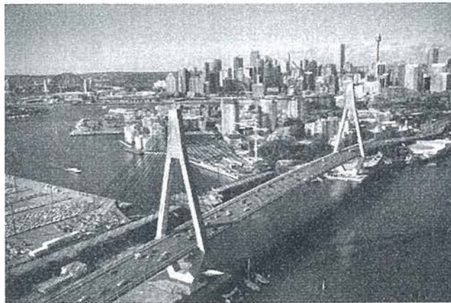
The ANZAC Bridge in Sydney is a cable-stayed bridge in which each cable forms a triangle with the pylons and the bridge deck.
